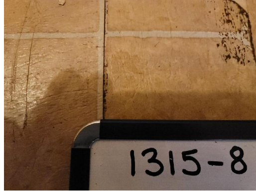
1315-8 12"x12" Floor Tile/Adhesive Bathroom (Top Layer) Living Room (Bottom Layer)
