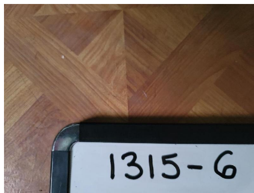
1315-6 12"x12" Floor Tile/Adhesive Interior Southeast Bedroom
