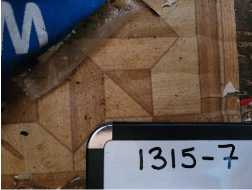
1315-7 12"x12" Floor Tile/Adhesive Northeast Bedroom
